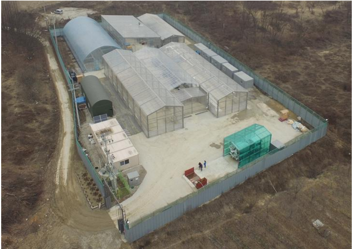
Fig. 1. Bird-eye view of the test bed for the SAFE research center. The test bed is an area of 6,500 square meters, situated on the finished sanitary landfill site minimizing public concern.
